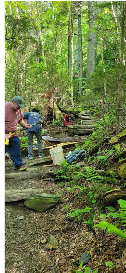
Randy Mitchell's crew doing some great work!
