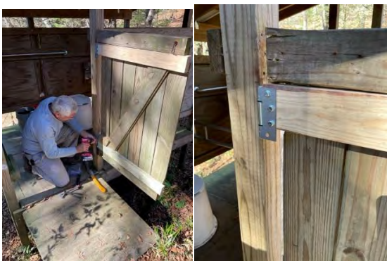
Bill replacing that hinge (photo courtesy of Taylor Weatherbee)
