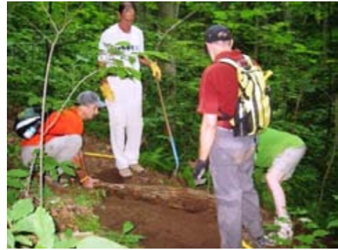
Sierra Club Workers leveling tread, repairing root ball and installing steps
