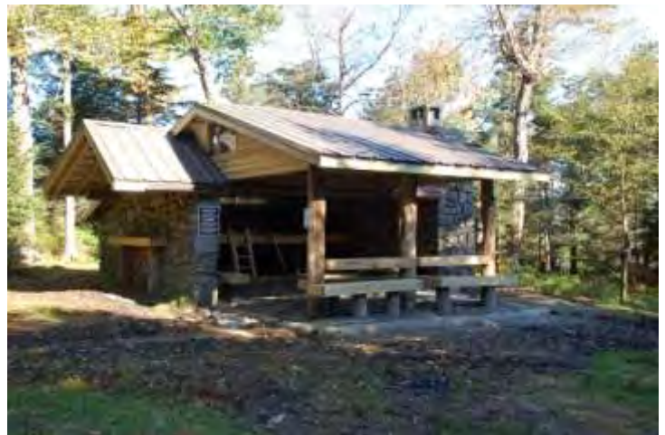
Mt. Collins Shelter Rehab, September 2009
