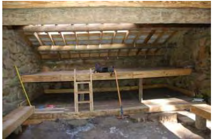
Mt. Collins Shelter Rehab, September 2009
