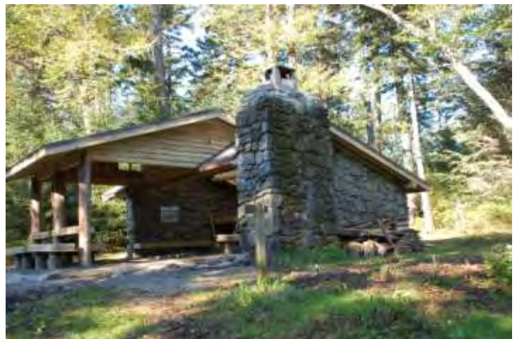
Mt. Collins Shelter Rehab, September 2009
